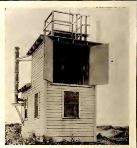
Above is shown a typical radio compass station, with the upper doors opened to show the loop mounted inside
