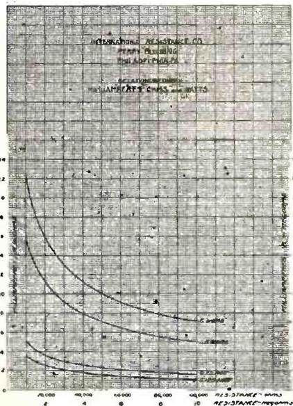
for milliamperes is taken from the left-hand margin, while if the resistance is considered in megohms, then the reading for milliamperes is taken from the right-hand margin.
