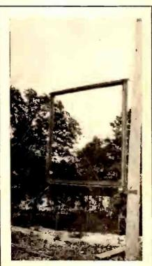
A double-beam radio beacon for aircraft
