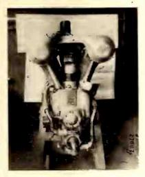
Showing ignition shielding installed on Liberty motor as means of suppressing noises in radio reception on aircraft
