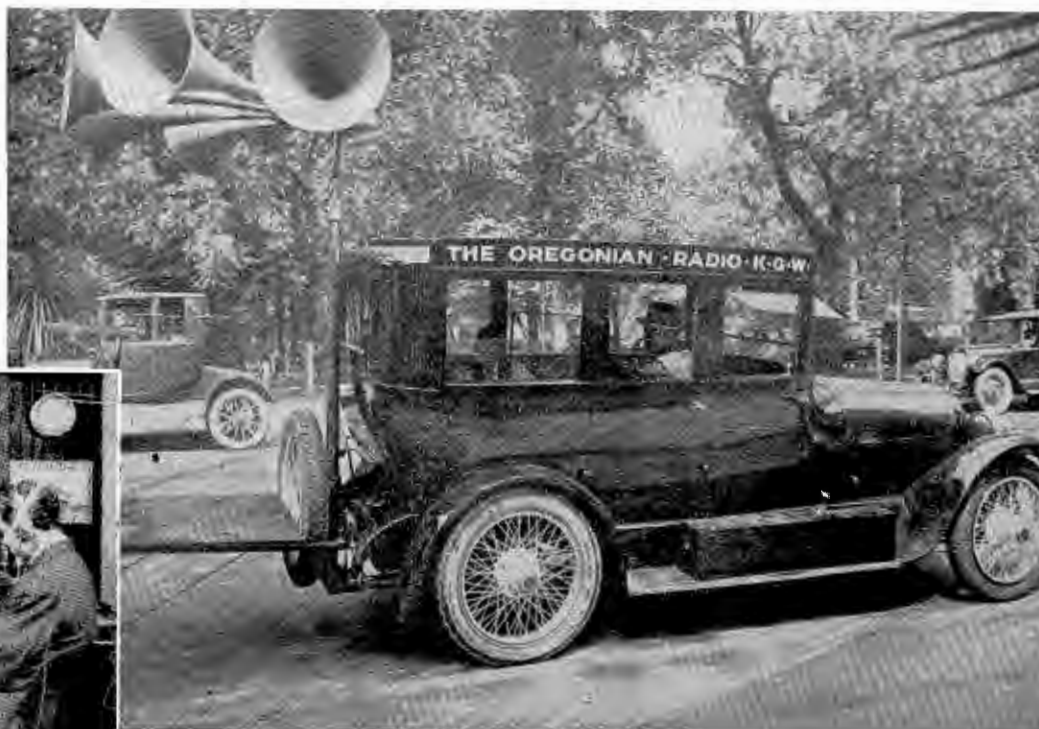
This is a far cry from the advantages of today's equipment. Reported to be the first remote and public address car used for radio. Taken in 1924 this car was in operation for The Oregonian Radio Station KGW in Portland, Oregon.
