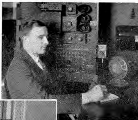
Herman D. Taylor, now plant manager and chief engineer at WTIC-TV-AM-FM, was chief operator for WTIC when this picture was taken in 1925 beside an amplifier rack in the station's control room. The transmitter could be operated by batteries when regular power failed.
