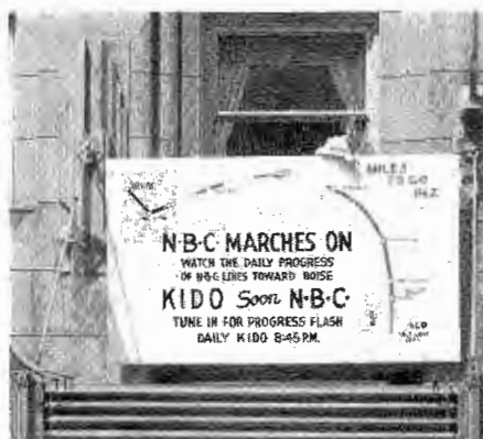
Mileage chart used by Station KIDO to bring NBC network into Boise, Idaho. 776 miles of copper wire had to be installed to bring the first network to Idaho. Line was completed and network programming began in Sept. 1937.
