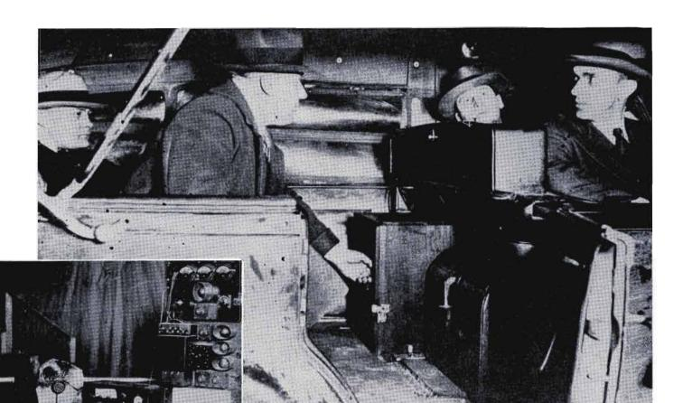
WGN radio's idea that led to the nationwide adoption of the use of radio receivers in police squad cars was given its first test in March of 1929 when the station installed radios in the cars of the Chicago Police force. Carl J. Meyers, engineering manager for WGN, Inc. is at the extreme left.
