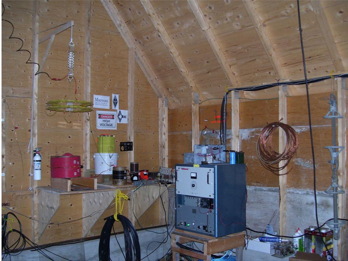
*Figure 5* Interior of the tuning hut, aerial tuning apparatus
