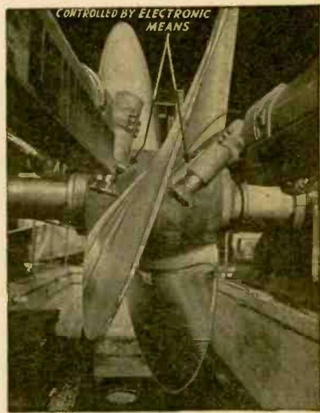
Propeller is shaped by large cutting burrs. Westinghouse Photos
