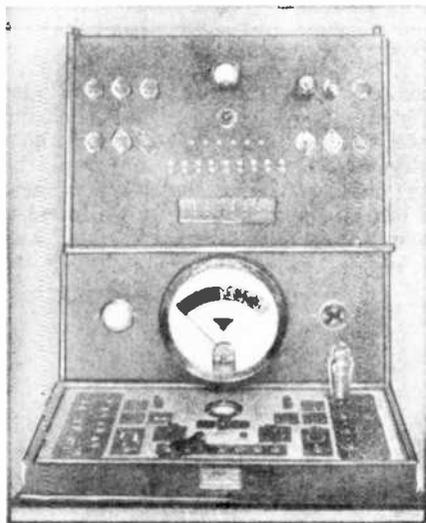
Fig. A. The infinite-resistance tube checker as operated in conjunction with a conventional tube tester. The leakage and resistance indicator is in the top center; below is the filament voltage selector switch. The 4 pin jacks are for point-to-point tube electrode checking (such as diodes). The 9 pin-jacks are also individual terminals and the numbers above them correspond to the respective socket terminals indicated about the left section of sockets. At bottom are the midget switches.
