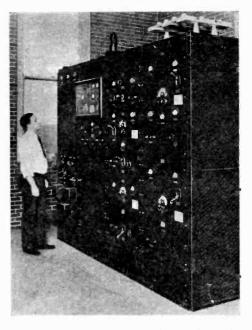
This illustration shows a section of the equipment recently installed in the new Westinghouse transmitting station of KDKA located near Saxonburg, Pennsylvania. This apparatus is for use with the short-wave transmitters. Shown in the photograph is the crystal control equipment, as well as the frequency multiplying and amplifying apparatus. This panel is of the very latest design and will insure accurate maintenance of frequency.
