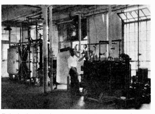
Fig. 1: A section of the condenser department, showing the large storage and impregnating tanks used in the manufacture of fixed condensers of various kinds.
