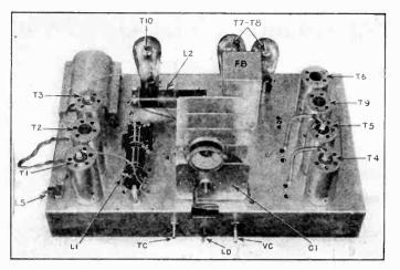
Left: The 10-tube Pilot super-heterodyne chassis with the coil shields removed. The various parts are lettered to correspond with the schematic diagram on bage 17. Below: the same chassis with the coil shields in place.
