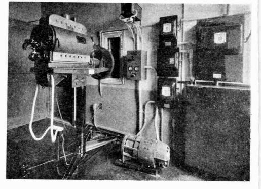
No, this is not a motion picture theatre projection room. It is the scanning room of the Columbia Broadcasting System's television station W2XAB. The heavy stand holds a 30-ampere arc light shining through a synchronously driven scanning disc, the combination producing a "flying spot" which travels over the face of the subject in the adjoining room. On the floor is the generator that feeds the arc.
