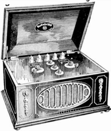
This Five-Tube, Couple-Circuit Receiver, utilizing both radio and audio amplification, in its present form represents the most advanced technique in the design of such sets. Has selectivity, sensitiveness and high quality of reproduction.
