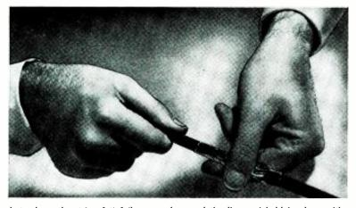
This photo shows the strip of tinfoil wropped around the line and held in place with a clip.
