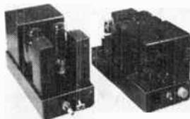
The amplifier is supplied with specially wound transformers and chokes and with capacitors of approved British Government type. It consists of two units, and weighs 47 pounds.
