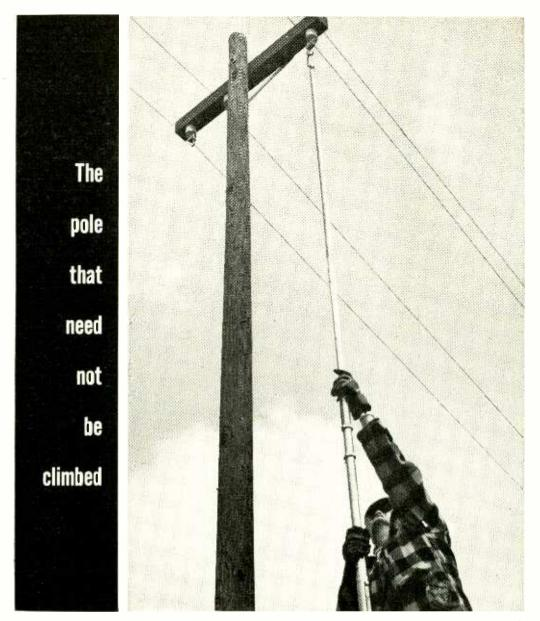
Fastening wires with new tool.
