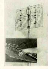
In addition to the adjustable dipole mounting bracket, there is side-by-side stacking of two 4-bay bows. The antenna has a sharp horizontal pattern which indicates a narrow beam width, and side lobes are negligible. The beam pattern of the major lobe width is 15° at the half power points, and average back rejection is 18 db.
