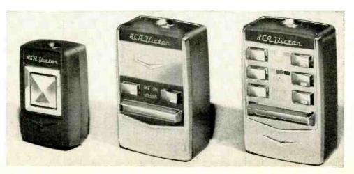
Three new RCA Wireless Wizard TV remote controls. On the left is 3-function unit for monochrome sets. Next is 5-function unit. At extreme right is new 7-function unit for color TV receivers.
