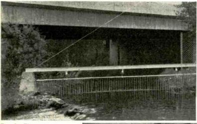
Fig. 2—Electrode system of an electronic fish screen at the intake for an irrigation district.
