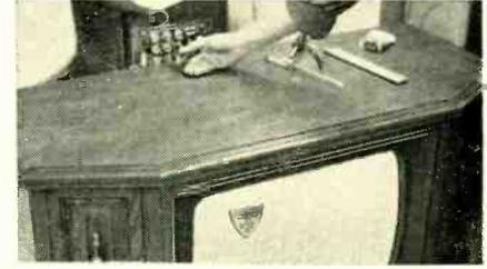
**TOP ROW, left to right. Loosen the screws that fasten the yoke assembly in place. Removing tube socket and blue-lateral magnet assembly. Convergence coils slip off tube neck.**
