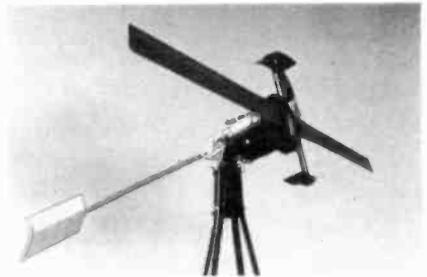
winds, delivers 15 amperes with winds at 23 miles per hour. Air-brake governor automatically prevents overcharging.
