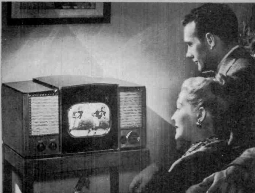
RCA's FAMED MODEL 530TS was television's equivalent to the model-T Ford automobile. The 530TS was the first post-war TV receiver and was also the first mass-produced and marketed TV receiver, selling for \$375.
