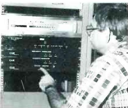
THE ACTUAL EQUIPMENT installation at WNYE-FM doesn't take up much rack space. Its Cue Page signal originates in a receiver that is tuned to WCBS.
