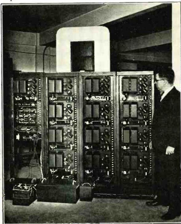
The giant public-address system installed in the three Chicago hotels housing the recent Radio Manufacturers Convention. The specially designed amplifiers were the product of the Samson Electric Company. The 150 speakers were Kylelectrons, the new condenser type, just introduced by United Reproducers Corp., and shown at the top of the picture.
