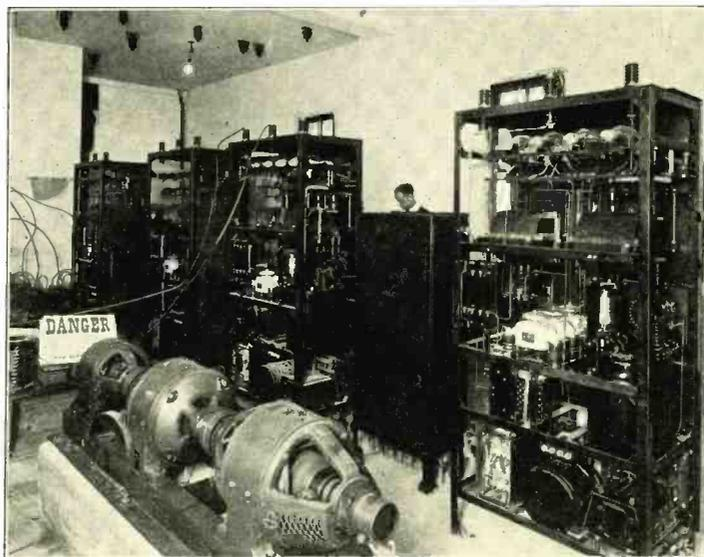
Fig. 20. Interior view of WJZ broadcast station, of the Radio Corporation of America, on 42d street, New York, installed in 1923. The station was designed to have simultaneous transmission on two wavelengths. The transmitting and modulating tubes may be seen on the top shelves of the power panels, of which a rear view is shown.
