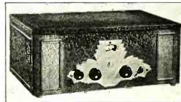
New Buckingham receiver, which has a tuned antenna circuit. It employs four 226's, one 227, two 171-A's in push-pull and a 280 rectifier. There is an adjustable hum control.
