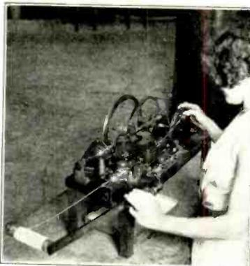
The Nucometer automatically and precisely measures, cuts, scrapes the ends and removes none of the oxide coating of filament wires. This machine—and it is one of two in the world—is used in the Duovac Radio Tube Corp., Brooklyn, N. Y.
