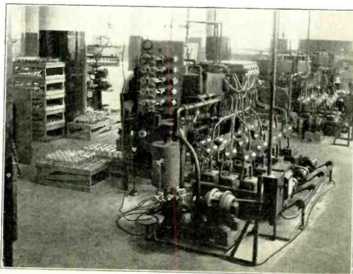
A bank of automatic evacuating machines in the Duovac Radio Tube Corp., Brooklyn, N. Y. The timing here is automatic and temperatures from 400 degrees above to 140 degrees below zero centigrade are used in this process.
