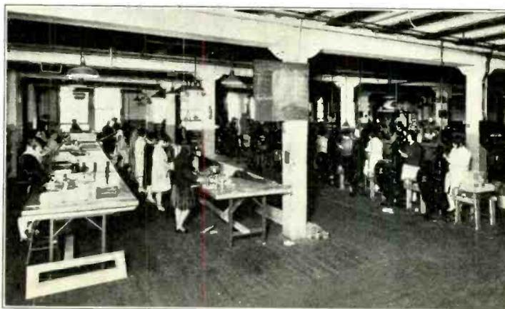
A portion of the Buckingham Radio Corporation's machine and assembly shop. Note the ample space and the special corrugated run-ways for hand trucks between the different groups. Female labor has been found to be highly efficient for this light work.
