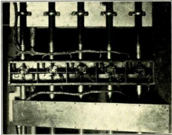
was found to be 0.0075 microhenrys per foot, the capacity 0.000456 microfarads per foot, and the approximate impedance 4.1 ohms.
