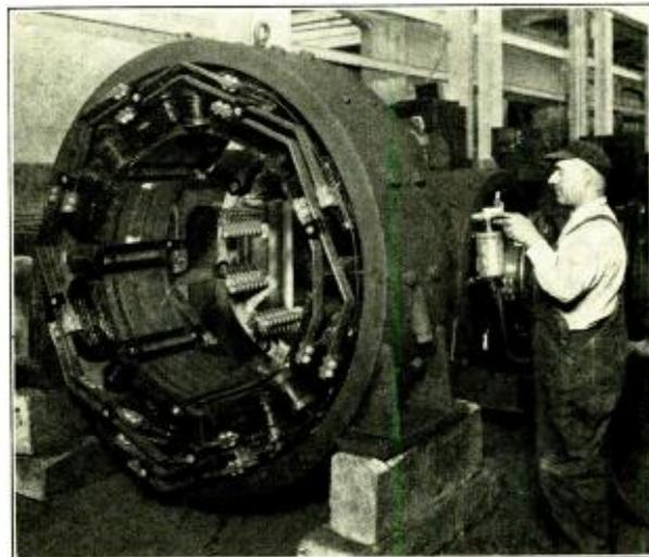
Factory application of Glyptal Lacquer on the frame of a d-c machine.
