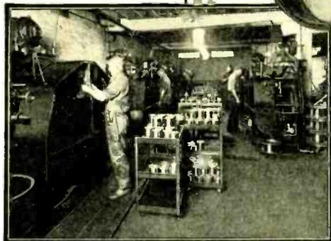
*Drawing bare wire through diamond dies to insure uniform diameter.*
