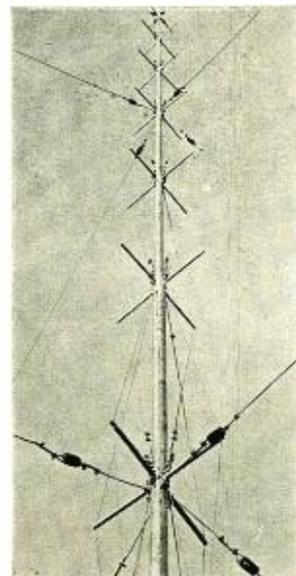
Fig. 2. Showing the wire cable trusses used to stiffen the steel pipe mast.
