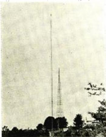
Fig. 1. View of the WMC reflector mast, and one of the vertical radiators.
