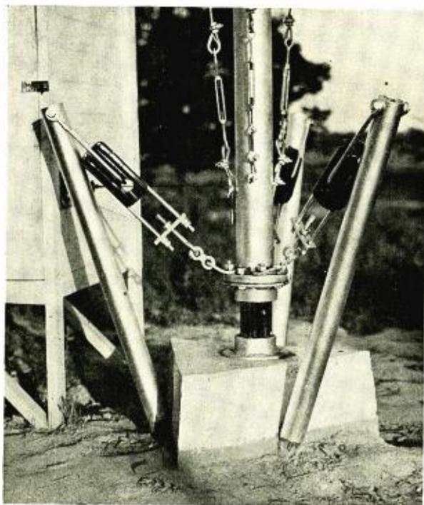
FIG. 3. VIEW OF BASE OF REFLECTOR MAST, BASE INSULATOR AND THE ANCHORAGE - LIFTING SYSTEM.
