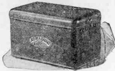
Trade Name—"Run-a-Radio"; Type—Bulb rectifier with filter circuit, use 2 bulbs to rectify both sides of wave; operates from 110 volts, 60 cycles, A.C.; delivers current for "A" circuit up to 9 tubes at 1¼ ampere each, "B" circuit up to 100 volts, and "C" circuit; replaces "A", "B" and "C" batteries; Material of Case—Metal, Gold crackle, enameled; Dim.—9 x 15 x 9 in. high; Weight—46 lbs.; Price—\$85.00.
