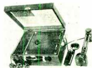
The Best Mfg. Co. has released the Model HRI home recorder, a portable, which uses an RCI control cabinet, an RMI microphone, and an RPI recorder pick-up. Compartments for necessary batteries are provided in bottom of the box. It is strictly an attachment for making recordings on pre-grooved composition records.
