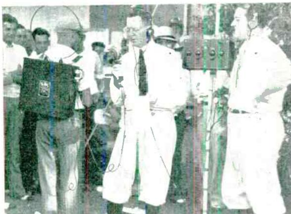
New portable short-wave transmitter and receiver used by NBC for field broadcasting.
