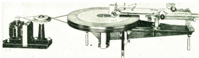
New Universal professional recording machine with 16-inch turntable and rim drive
