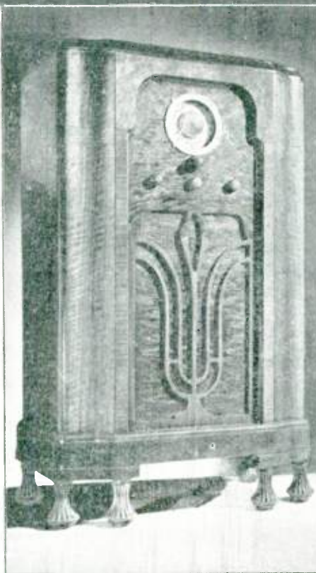
★ (Above) 7-tube Ferrodyne receiver with all metal tubes. New Diffusalite Magic Dial. ★
