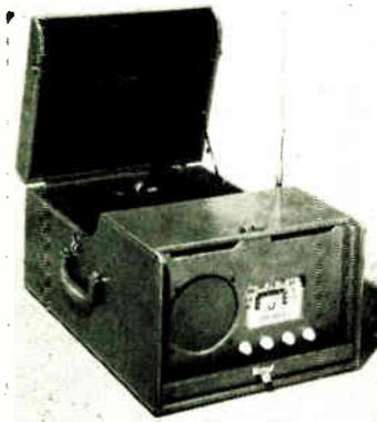
Among the important features of this machine, which is in the luxury class, are a collapsible short wave antenna, a Magnavox speaker, a push-pull tone system. It has seven tubes plus rectifier, pre-selected R. F. stage, and is built to operate up to 220 volts. Finished in top grain suntan cowhide or aero-tweed.
