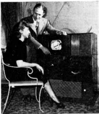
Stan Glaser, manager of radio and television for the Crosley Division, Avco Manufacturing Corporation, demonstrates the "Swing-A-View" picture tube in the new Deluxe Spectator television receiver. The three-band radio and phonograph console was introduced publicly for the first time at a press preview at the Hotel Waldorf-Astoria last month. Unique feature of the "Swing-A-View" is the picture tube which may be viewed from any point along a 60-degree arc in front of the receiver.
