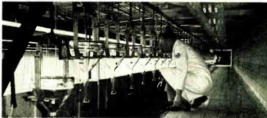
*This view of gleaming glass blanks at RCA's Lancaster plant is typical of television manufacturing. Automatic machines pass glass bulbs from process to process until they emerge as cathode-ray picture tubes for TV receivers.*
