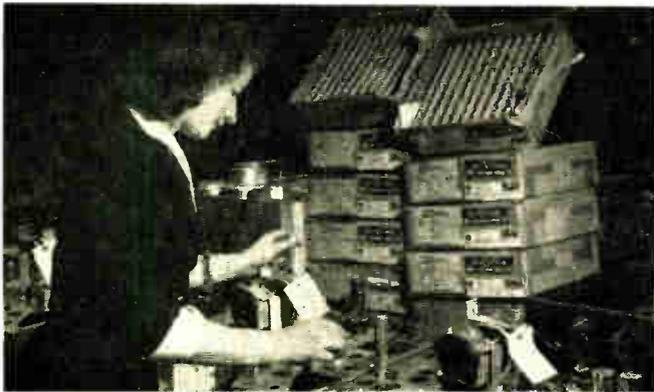
Deflection yoke and bracket are followed by electron tubes during chassis' 2000-foot conveyor belt ride.
