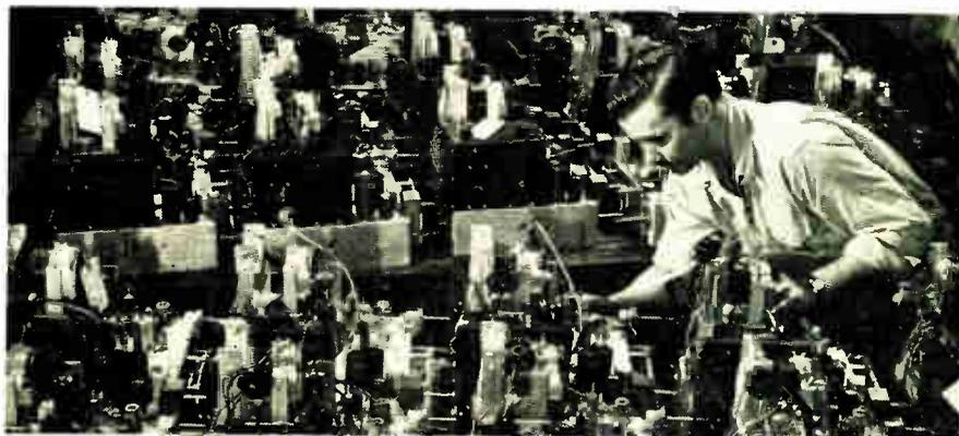
*Television chassis are intricate pieces of mechanism. Receivers have from five to six times more tubes than the ordinary radio set. An inspector like the one above must test each chassis before passing it along to cabinet assembly.*
