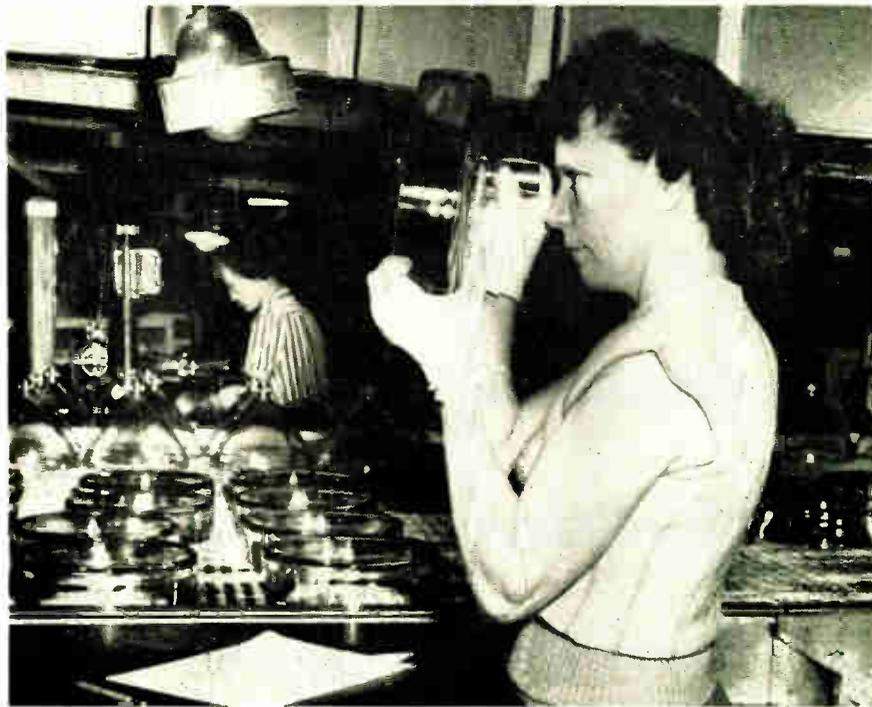
*Glassmakers had to convert from hand to mechanical processes to lick television picture tube bottleneck. This girl sees to it that face plates going out of Kimble Glass plant of Owens-Illinois Glass Company are flawless.*
