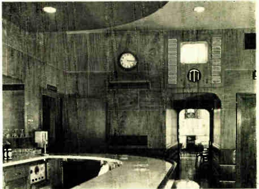
**Note multiple viewing units in this television arrangement. Screen above the door is designed to fit in with woodwork. Second viewer is in side room beyond. Remote control unit is behind the bar to left.**
