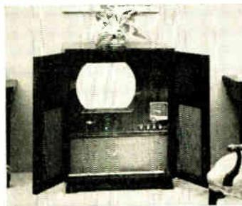
To give its 203 square inches of picture space, this television console uses the new short-necked 19-inch cathode-ray tube. Instrument contains full-range FM radio and plug-in receptacle for record player. Has firm's local-distant switch and two-speed square selector dial. Set has 25 tubes and five rectifiers. Cabinet is made of mahogany veneers.
