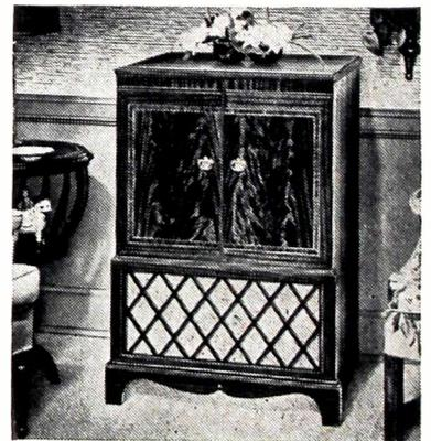
Heading this firm's 1951 line is this console TV receiver which features a 17-inch rectangular picture tube. For greater convenience, the phono-switch is located on the front, combined on the instrument panel with the tone control. Set stands 36¾ inches high, is 28 inches wide and 23 inches deep. Price, in walnut or mahogany, \$389.50.
