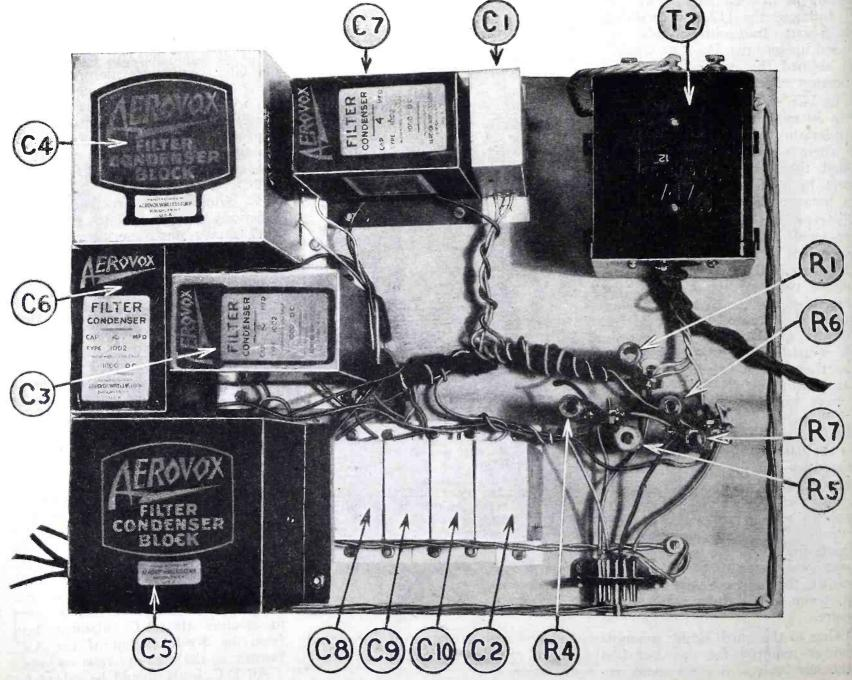
A bottom view of the completed Home Concert Amplifier showing how the condensers, fixed resistors and cable-plug connector are mounted and wired.
