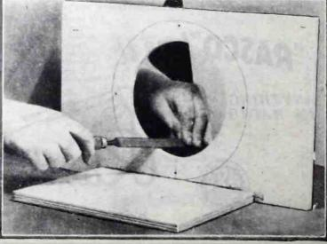
Fitting and filing the hole in the baffle.
