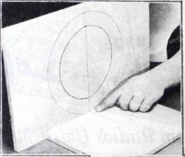
popularity, requires a baffle board for its most satisfactory operation. This baffle is merely a plain board about three times the area of the mouth of the speaker, with a hole cut in it to accommodate the latter.
