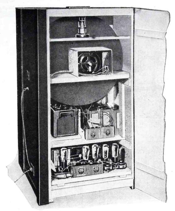
A rear view of the television receiver showing the universal motor which drives the scanning disc. Above the motor is the Moore neon lamp. On the lower shelves are batteries and the amplifier and rectifier tubes.
