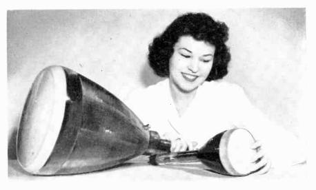
Two RCA Cathode Ray Tubes of the type used in television receivers.
