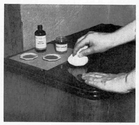
Fig. 8 Finishing by the Dip and Rub method. An excellent finish which is somewhat easier to obtain. It is not quite as fine as a French finish but is entirely satisfactory.
