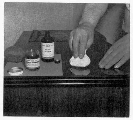
Fig. 7 French finishing. By using French Varnish and Emulsion and applying it as shown, a very fine finish can be obtained.
