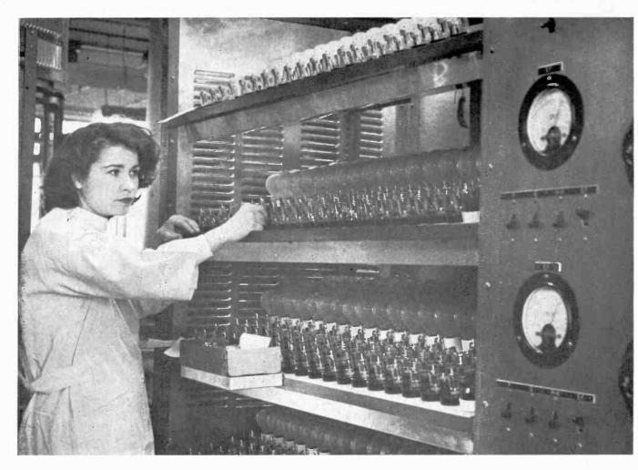
A pretty tube plant worker watches miniatures being aged on a rack. The ageing process, which stabilizes tube characteristics and eliminates
