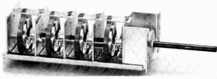
The four-gang "Inductuner." Note mechanical simplicity of this unit, which is a basic tuner for front-ends built by several companies in addition to Mallory. Shorting fingers and spiral inductances can be seen in this picture.
