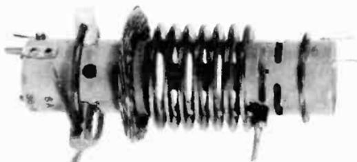
Figure 148. An r-f supply transformer.
