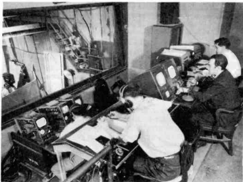
Figure 18. The studio control room. The technical director is seated before the switching console. (courtesy WPIX)
