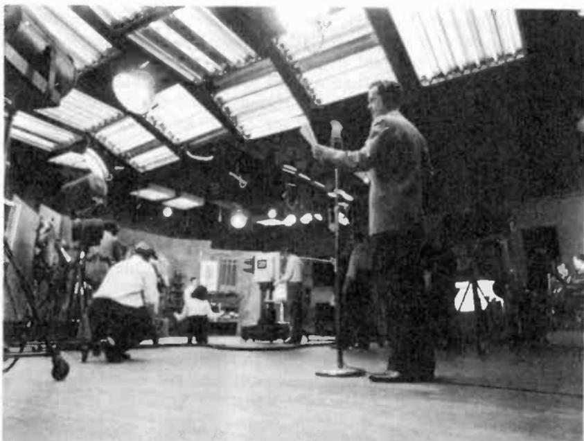
Figure 8. A studio equipped with fluorescent lighting.
