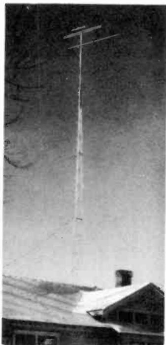
Figure 26. Lightweight tower for mounting television antenna.
