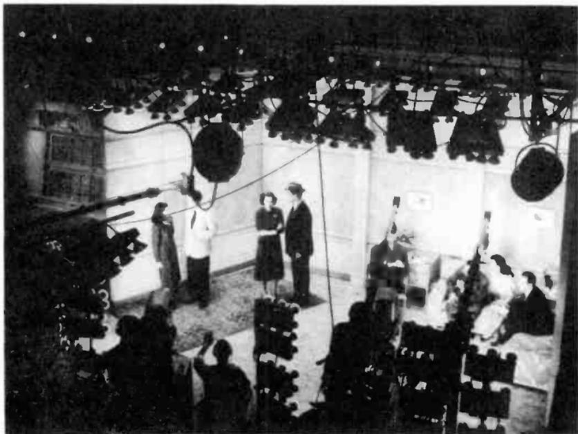
Figure 7. Large banks of lights are necessary with iconoscope cameras. (courtesy DuMont)
