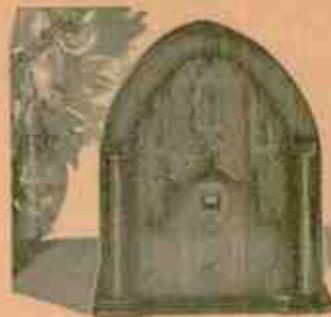
**THE HAMILTON** — 4-tube AC Superheterodyne Receiver. 110 volt, 60 cycle current. Available to operate on 110 volt, 25 cycle current or 220 volt, 50 cycle supply. Superheterodyne circuit . . . dual wave. Frequency range broadcast band 550 kilocycles to 1500 kilocycles. Police band 1400 to 3400 kilocycles. Tone control . . . colorfully illuminated dial. Tube complement 1-6F7, 1-75, 1-75, 1-42, 1-90. Beautiful Gothic cabinet. Height 13 1/2", Width 11", Depth 8 1/2".
