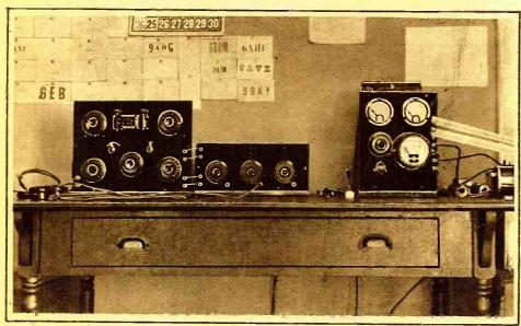
This Station Is Neat In Appearance Due Particularly to the Absence of Unsightly Wiring. I and Long-Wave Receiver Is on the Extreme Left Followed by the Detector-Amplifier Unit.
