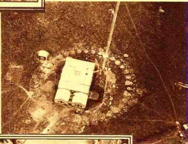
**BIRD'S EYE VIEW OF 5XX.** This photograph, taken from the top of one of the 500-foot antenna masts, shows clearly the ring of thirty-five ground plates surrounding the station. The lead-in from the antenna may be seen in the middle of the picture.
