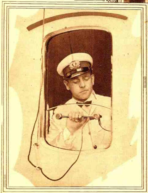
NOVEL LEAD-IN ON SHIPBOARD. To bring the lead-in through top of the window would prevent its being closed, so the operator fastened the wire to each side of the handle that is used to raise the glass and so successfully solved the problem. © Kadel & Herbert.
