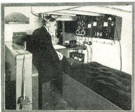
Interior of wireless cabin, showing Radio Operator Gilbert Moss, seated before his instruments. Behind him, on the deck, is the loop antenna, unshipped. In the corner of the bench is the ¼ K.W. quenched spark transmitter, and on the bulkhead in front of Mr. Moss is the 6-tube radio compass receiver and the 2-tube all-wave receiver, both fitted for alternative crystal operation. Photos © Marconi Wireless Telegraph Co., Ltd.
