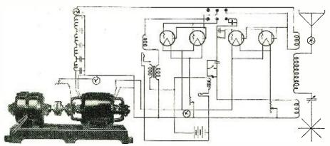
There is no question about the Miles per Watt with ESCO-it is the maximum. Item 35. Two unit four bearing set. Furnished with ring oiled or ball bearing Motor to suit local supply. This "ESCO" set delivers 1000 volts, 300 watts for plate supply and 12 volts, 150 watts for filament supply. This set driving two 50 watters will make a good
