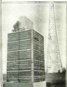
WATER COOLER FOR VACUUM TUBES. This huge water cooler, which is capable of cooling 100 gallons of water per minute, is used for the purpose of keeping the giant vacuum tubes used in the transmitter at an operating temperature. This is necessary because the great power which is needed to operate these tubes would ruin the comparatively delicate elements in a short time.
