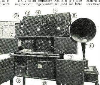
The 23-control radio set assembled by Mr. Silverman. The component parts are numbered in accordance with the text.
