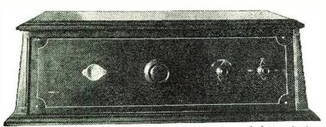
The receiver described below has an unusually harmonious appearance, as the front panel and knobs are made of wood to match the rest of cabinet. All metal work is lacquered brass. The dial is illuminated from the rear by a small bulb (shown as No. 7 below).
