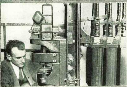
A MOTOR - OPERATED OIL SWITCH. Above is shown one of the large switches, which is located in a house of its own and controlled es, which is located in a houseof its own and controlled
