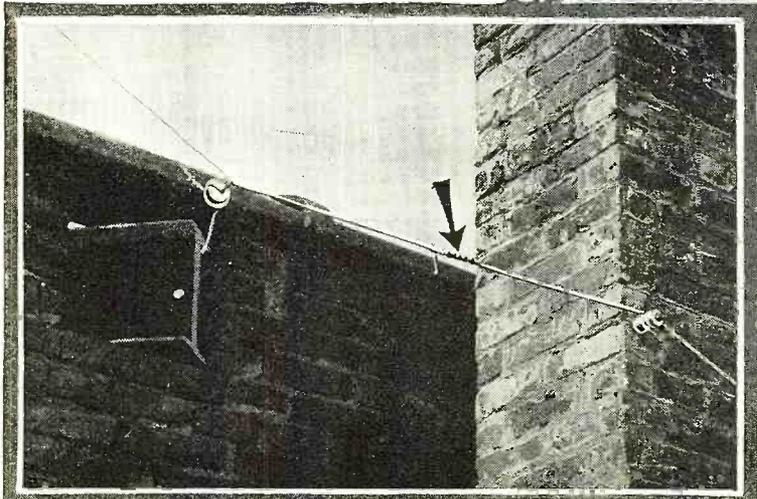
This aerial is well insulated from surrounding objects and is securely fastened. However, the lead-in is merely twisted around the aerial wire instead of being soldered thereto.
