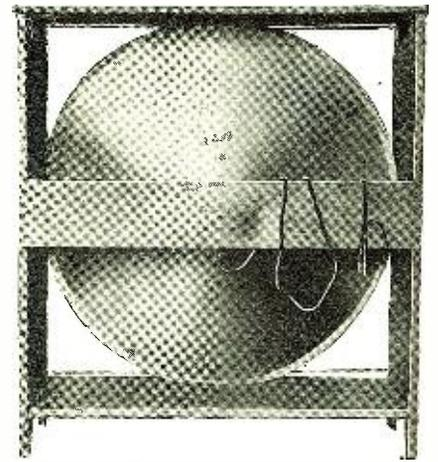
A rear view of the completed cone speaker. The unit is mounted on the wooden cross member. Photo courtesy of Engineers' Service Co.
