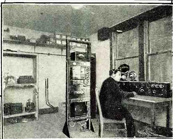
One of WRNY's operators is shown making a preliminary adjustment upon the transmitter. The wavelength of this is varied by the condenser and variometer controls shown.
