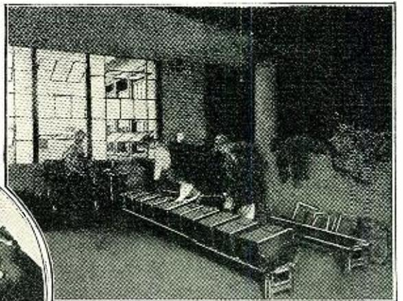
One of the batteries of electric furnaces, each capable of maintaining a temperature of 5200 degrees Fahrenheit, used in the melting of silica sand, and the amalgamation with it of reducing materials and several alloys used in manufacturing silite, the new metallic glass-like rectifying element, which takes the place of precious metals by its resistance to acid.
