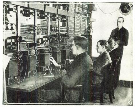
The WEAF control board, located at 195 Broadway, New York City, through which all the chain broadcasts over the "Red" network are distributed.
