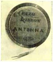
Cellophane covering may be had in a variety of colors, harmoniously adapting the antenna to the decorative color scheme at hand. This new type of ribbon antenna is flexible and can be fastened around mouldings or baseboards without difficulty. comes in standard lengths of 50 feet and
