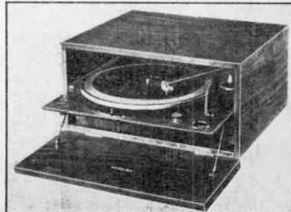
to permit adjustment of the record and the pickup. It is equipped with a volume and a speed control and there is a special lever attachment on the pickup to facilitate placement of the record. It employs a 12-inch turn-table. The attractive walnut cabinet measuring 9 by 15 by 17 inches is ideally suited both for size and style for placement below a midjet radio or on top of a console. It is available for a.c. or a.c.-d.c. operation.
