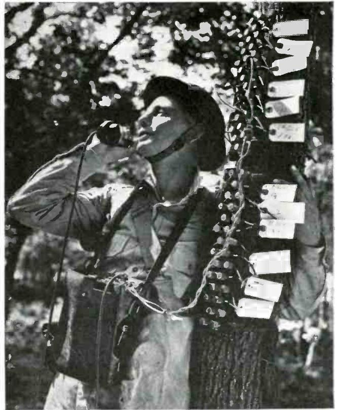
Signal Corps student operating a field telephone test station. Tags identify various lines extending to many field divisions.
