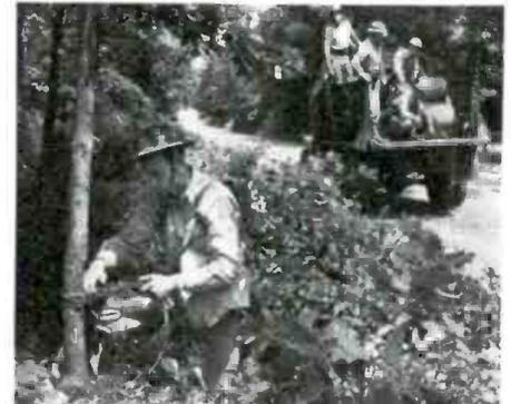
A Signal Corps lineman tying field wire in place prior to stringing.
