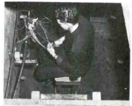
Birdseye view of student at work in manhole making wire cable connections.
